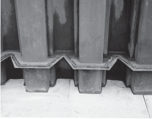
Fig. 2.1. Welded horizontal plates with hydrophilic strip.
