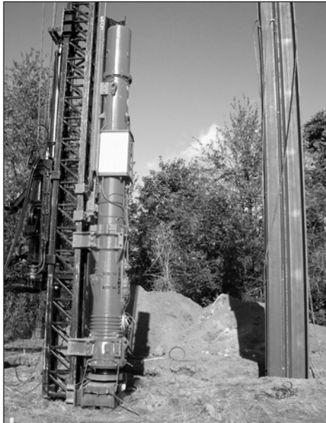
Fig. 11.6. Diesel hammer on fixed lead.
