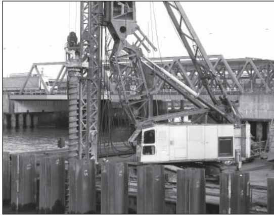
Fig. 11.26. Predrilling for a combined wall installation.
