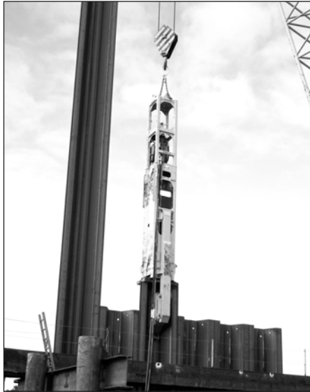
Fig. 11.8. BSP CX85 driving AZ piles.
