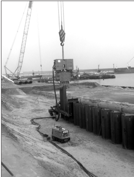
Fig. 11.10. Rope suspended HFVM vibratory hammer.
