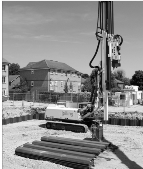
Fig. 11.13. Telescopic rig with vibratory hammer.
