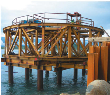
1. Installation of template
