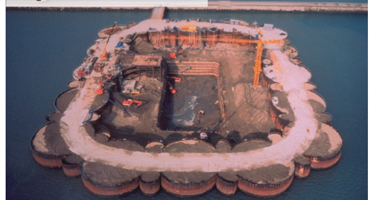
Bridge construction, South Korea
