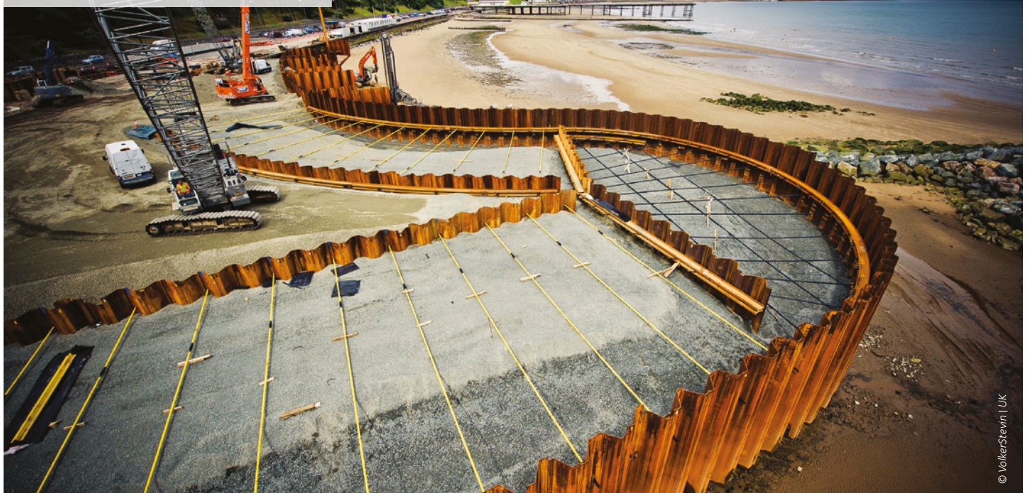
Coastal defense project, Colwyn Bay, UK
