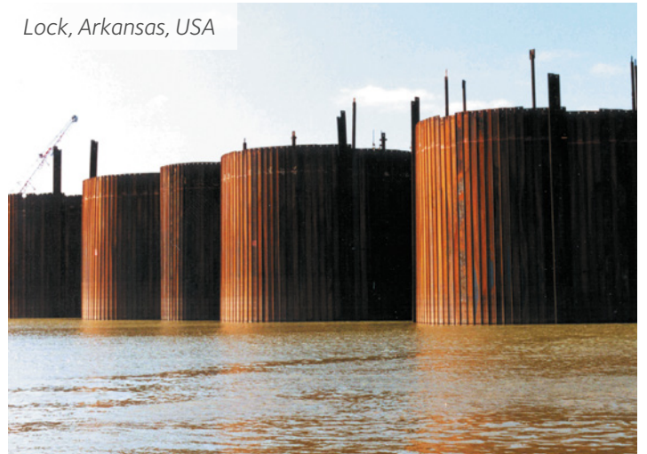
Diaphragm cells with 120^\circ junction piles.
