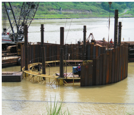
2. Threading until cell closure
