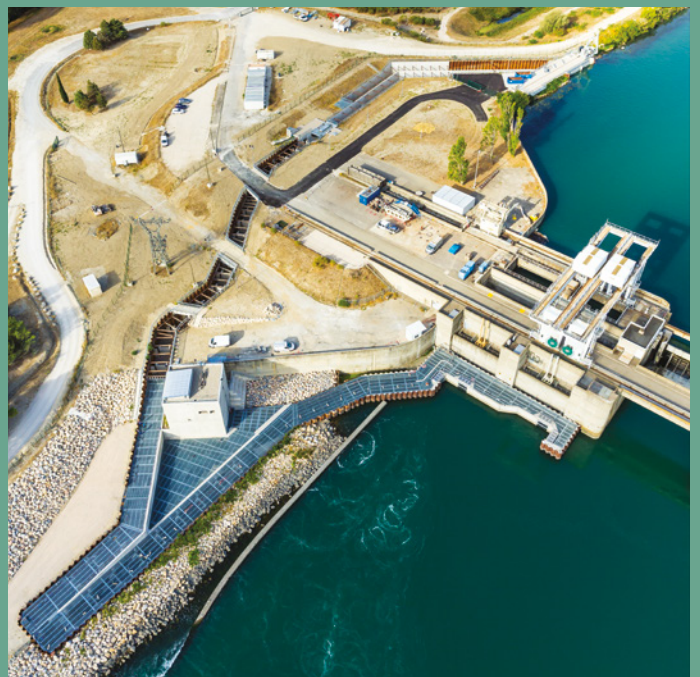
Fish pass at Sauveterre hydroelectric dam on river Rhône, France, allowing the restoration of the migration path of several fish and wildlife species. © Juan Robert
