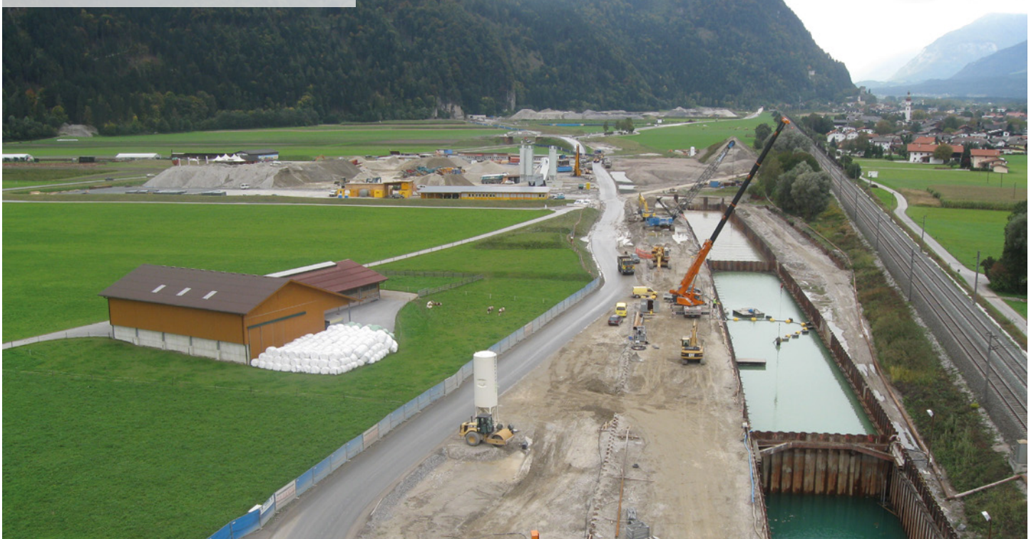
Temporary trench, Brenner railway, Austria
