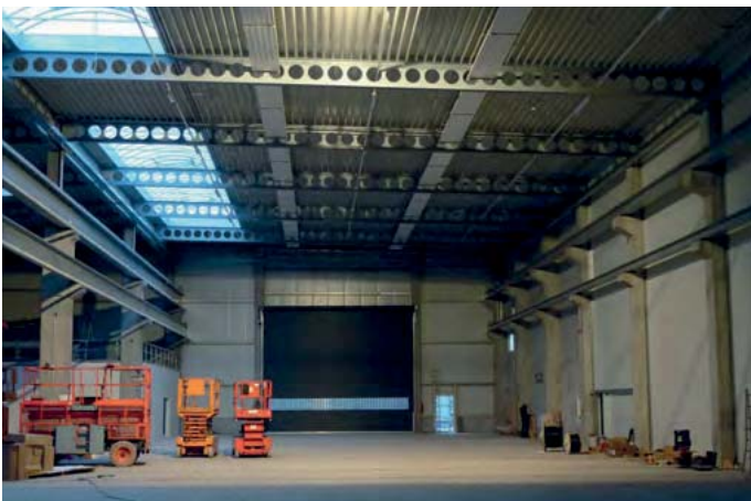
Figure 2: ACB® roof beams
