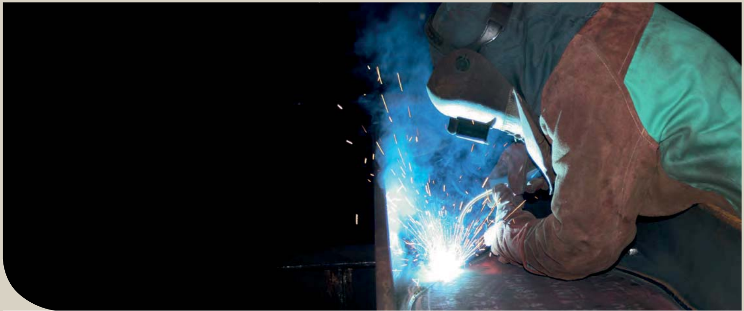
Figure 7: Fabrication of Angelina® beams
