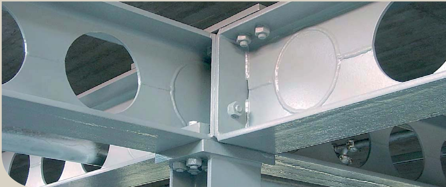
ACB® beam featuring filled openings at support
