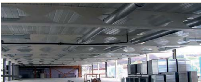
Figure 24a: Angelina® beams in composite floor systems
