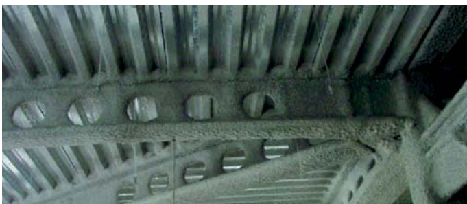
Figure 27: Protection by spraying on ACB® beam
