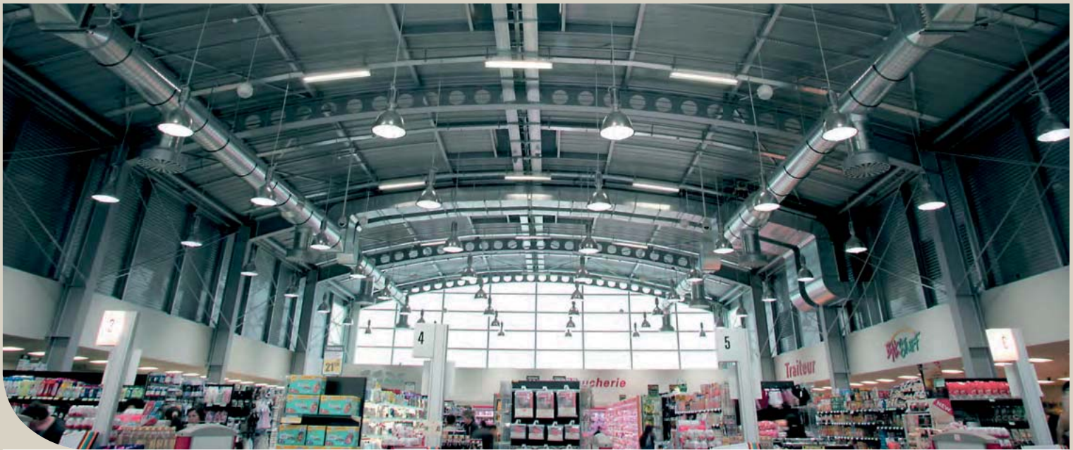
Cellular beams spanning 25 meters and featuring important camber
