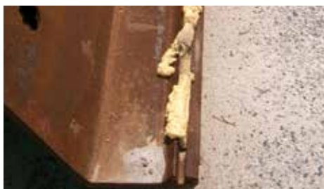
Closing interlocks with foam or grease
