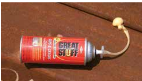
Closing interlocks with foam or grease
