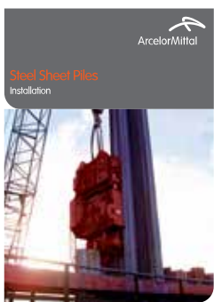
Installation of sheet piles GB, DE, FR
