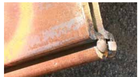
Bolt inserted in leading interlock
