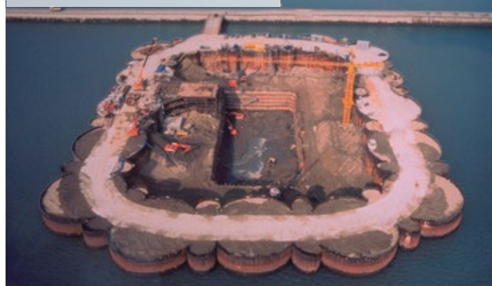
Bridge construction, South Korea
