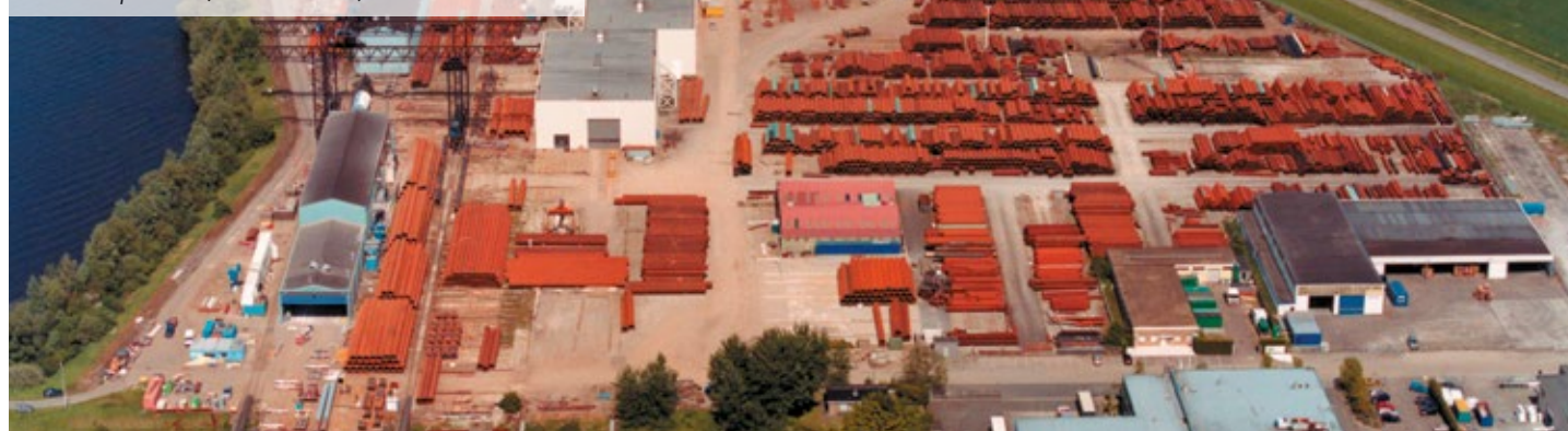
Tubular pile mill, Dintelmond, The Netherlands
