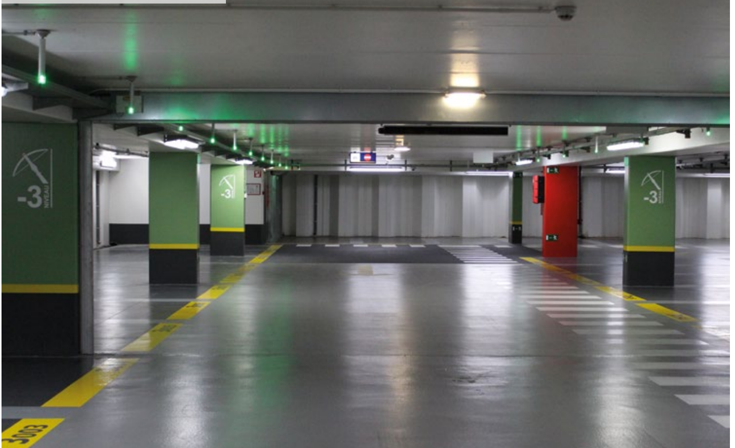
Underground car park, Aalst, Belgium
