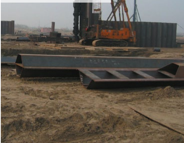
Changxin dry dock, Shanghai, China
