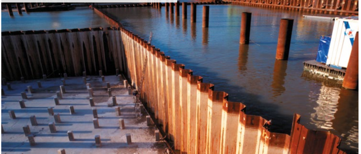
Excavation for an office building, Amsterdam, The Netherlands
