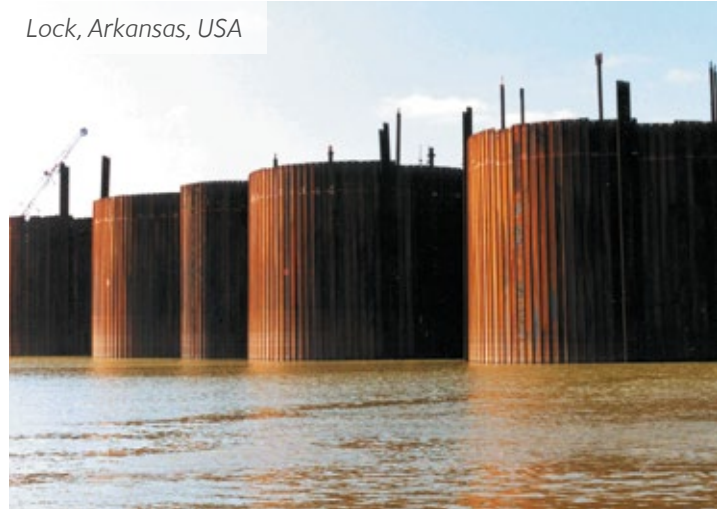
Diaphragm cells with 120^\circ junction piles.
