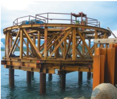
1. Installation of template
