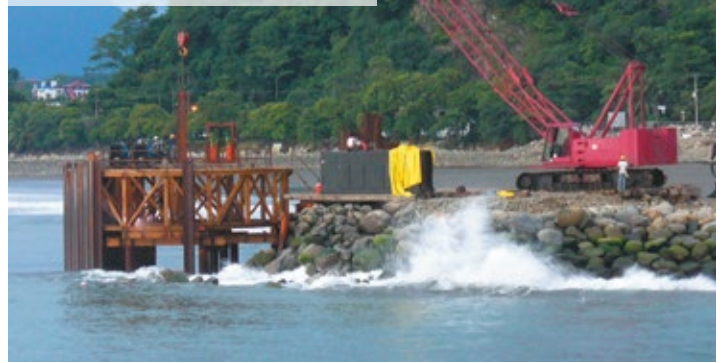
Marina breakwater, Costa Rica
