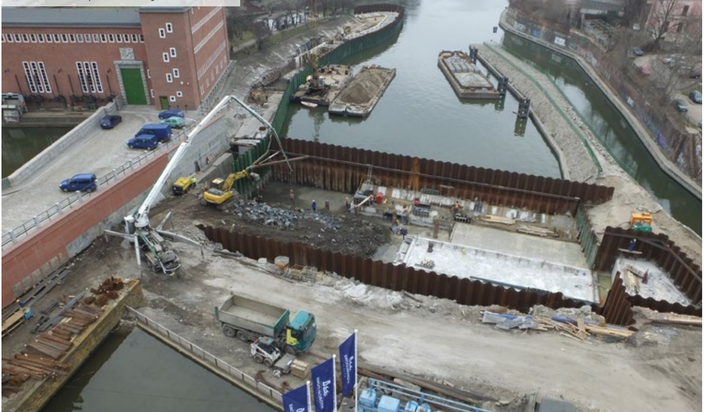
Wroclaw flood protection system, Poland
