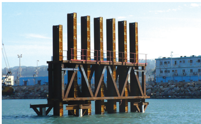
Fig. 9. Driving templates and their support.
