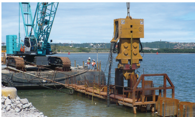
Fig. 10. Template and detail of guide.
