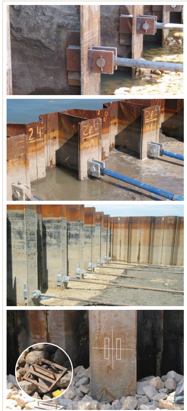
Fig. 5. Installation of the T-connectors at the job-site.
